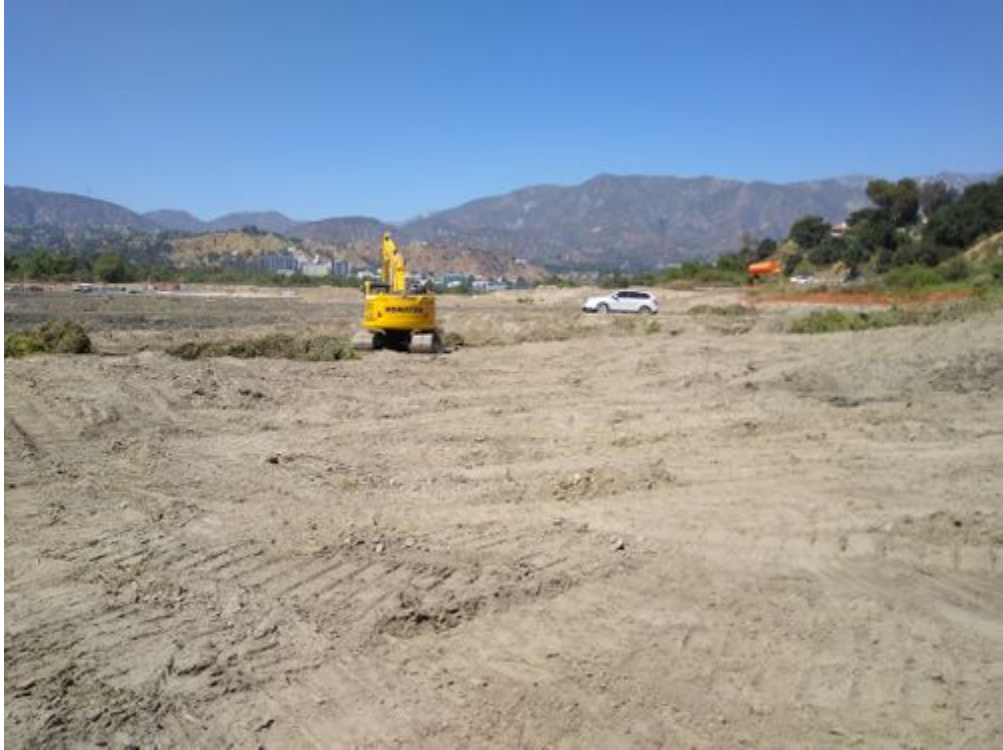
photo_3-work area post removal.jpg -118.17427 34.18635
