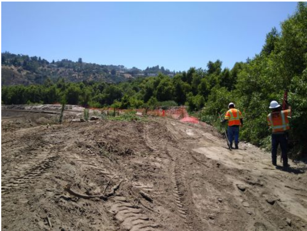
photo_4-ESA fence restoration.jpg -118.17598 34.18923
