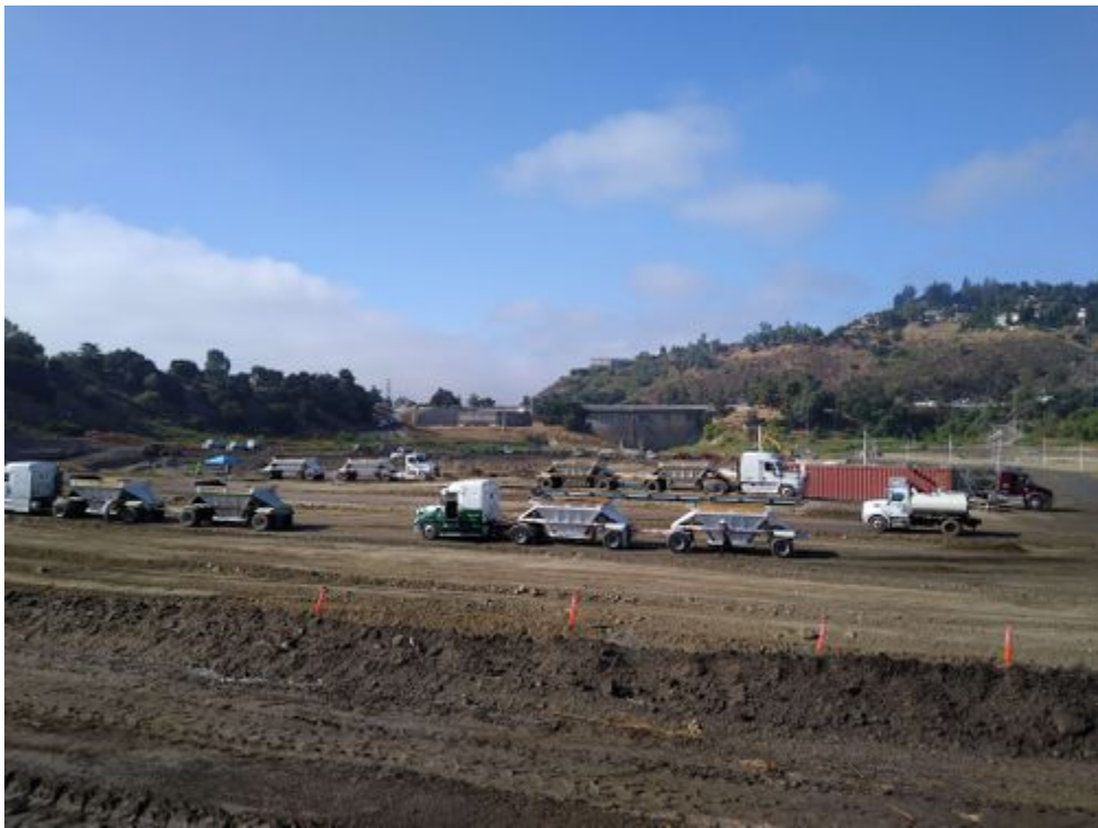
Photo_2-sediment removal activities.jpg -118.1745 34.18983
