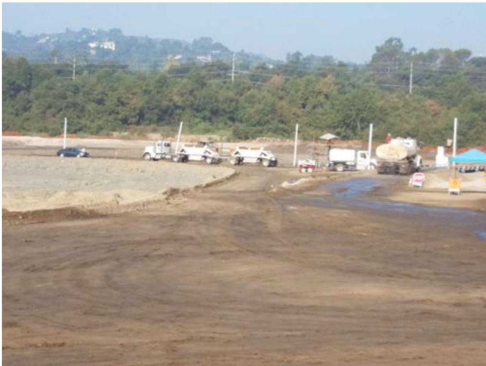
photo_2-20200921_sediment removal_facing W.jpg -118.17348 34.1888
