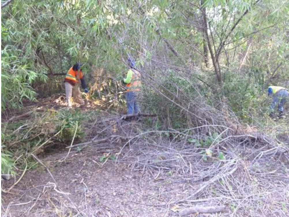
Photo 1-weeding in progress, DG-4, facing NW.jpg -118.17736 34.18906
