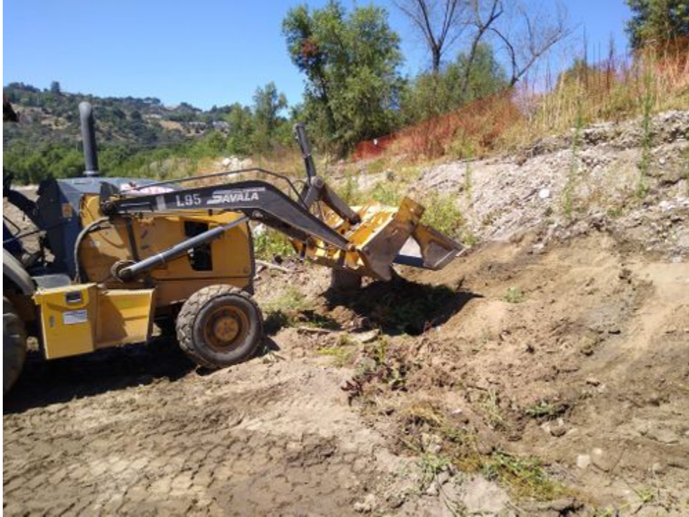
photo_3-vegetation clearing west of scalehouse.jpg -118.17535 34.18974
