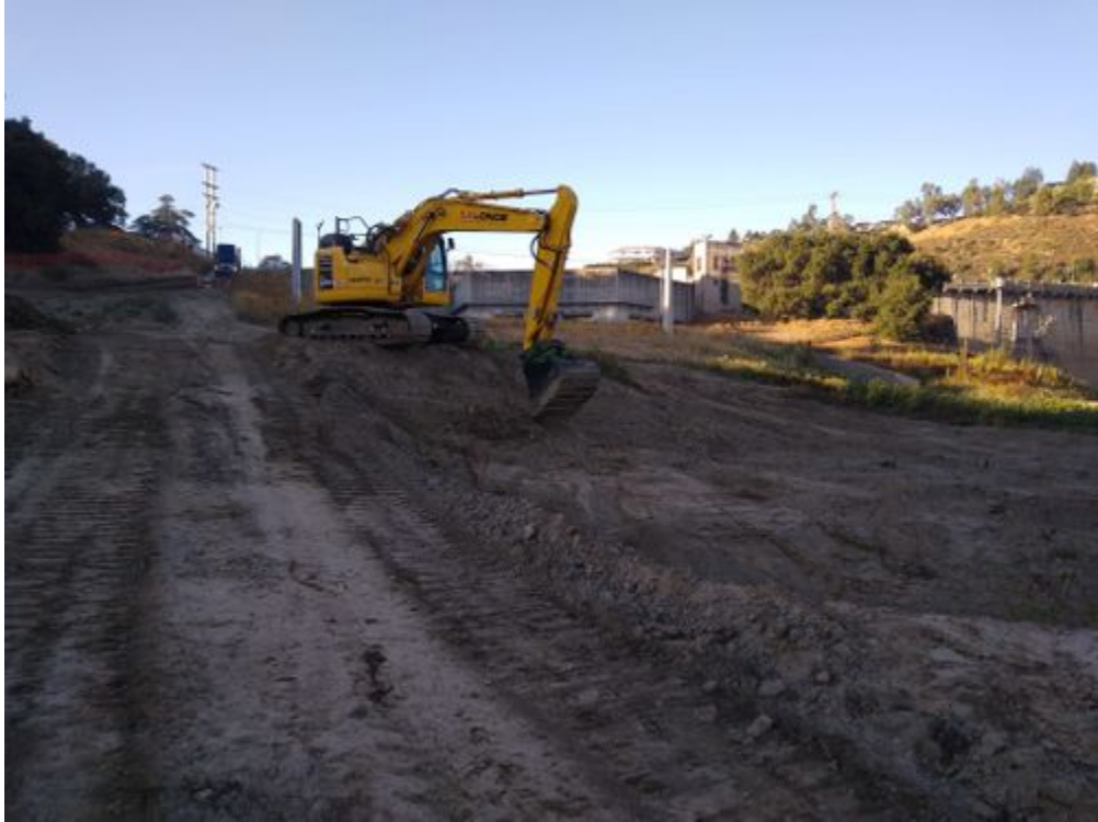
photo_1-excavator removing vegetation piles.jpg -118.17396 34.18673
