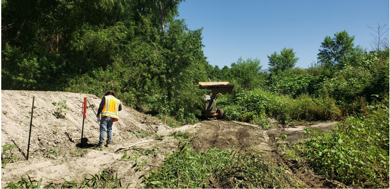
Vegetation clearing for fence reinstallation on west side.jpg
