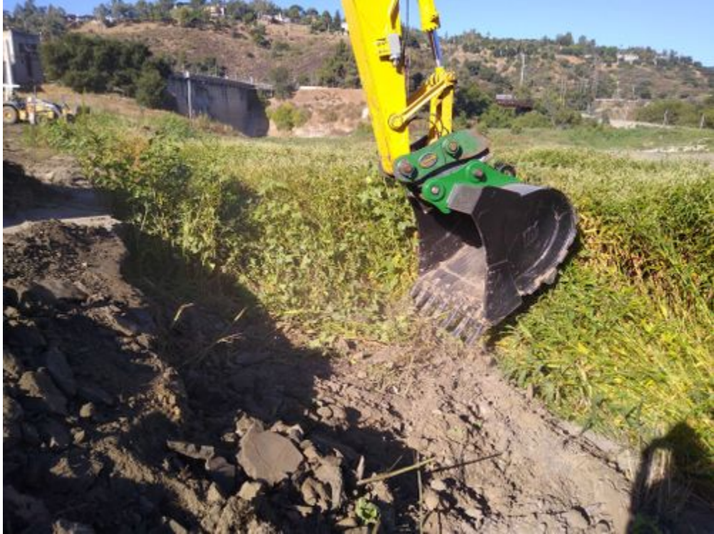
photo_1-excavator clearing vegetation.jpg -118.17369 34.18681
