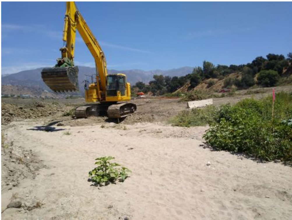
photo_2-excavator removing vegetation.jpg -118.17496 34.18601
