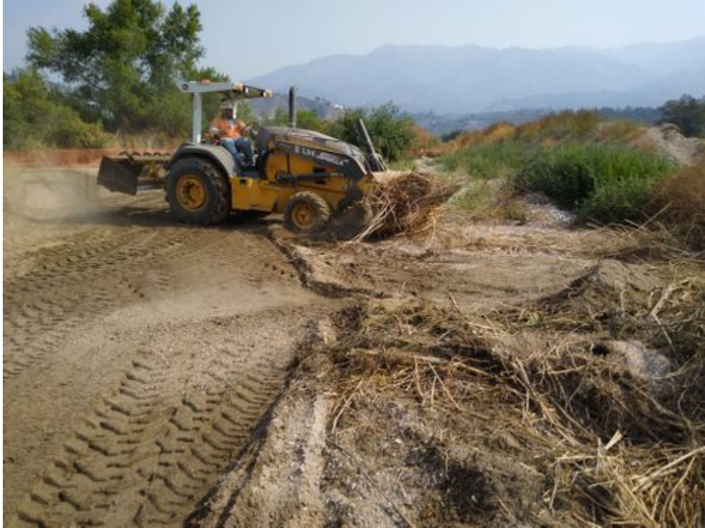
photo_1- vegetation removal.jpg -118.17272 34.19226
