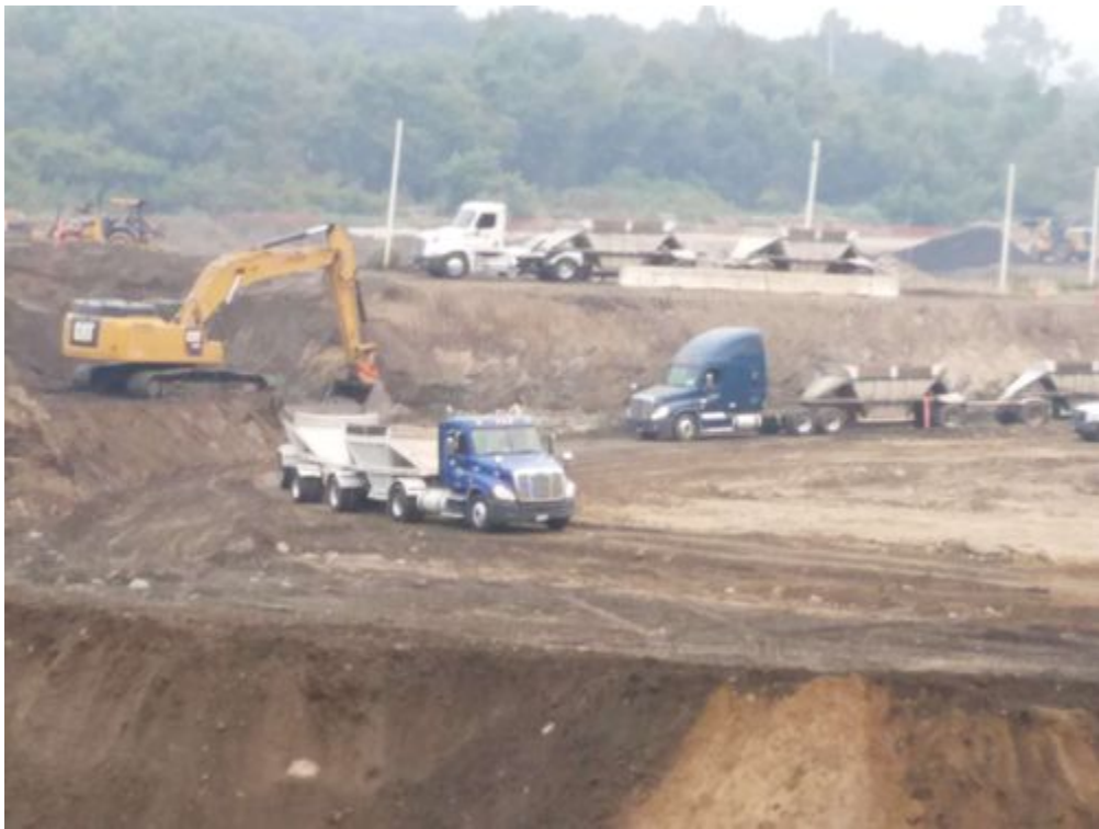
photo_2-sediment removal_facing NW.jpg -118.17484 34.18589
