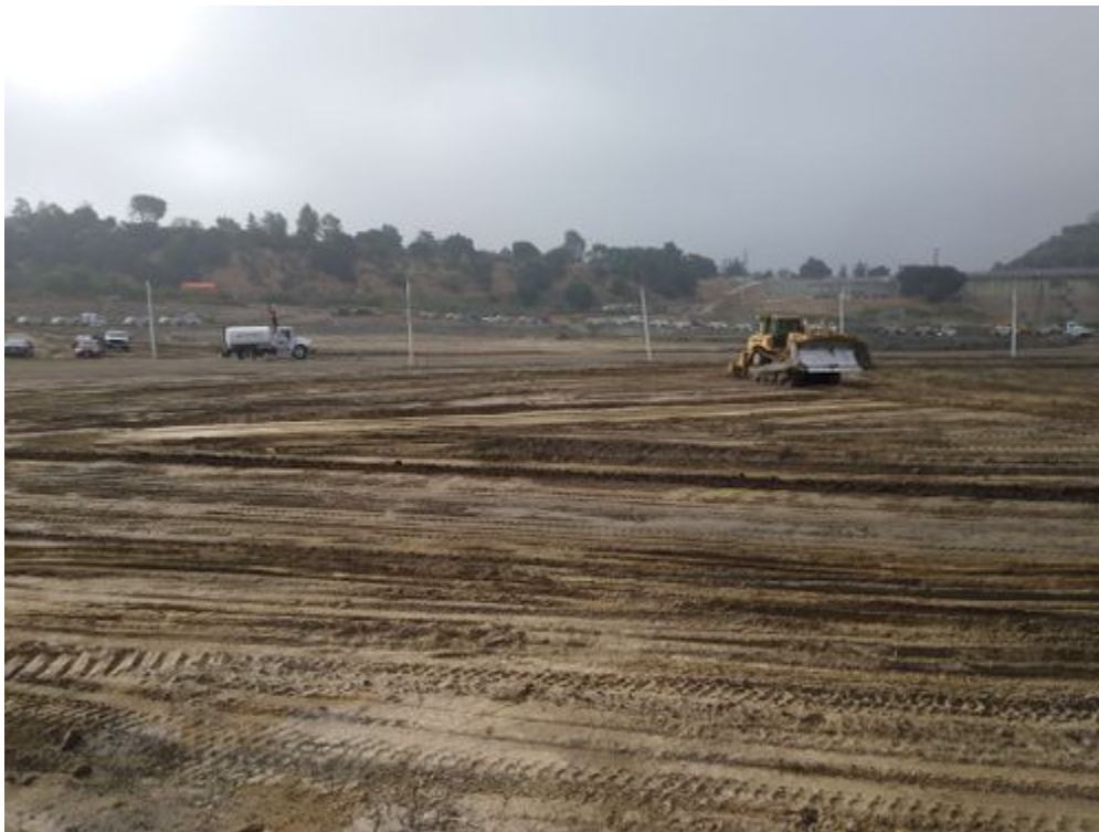
photo_2-sediment hauling activities.jpg -118.17565 34.18935
