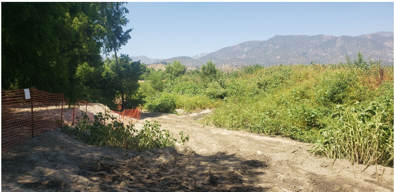
After vegetation clearing and fence reinstallation on west side.jpg
