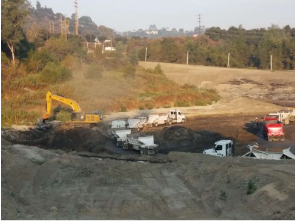
photo_1-20200918_sediment removal_facing W.jpg -118.17437 34.18601
