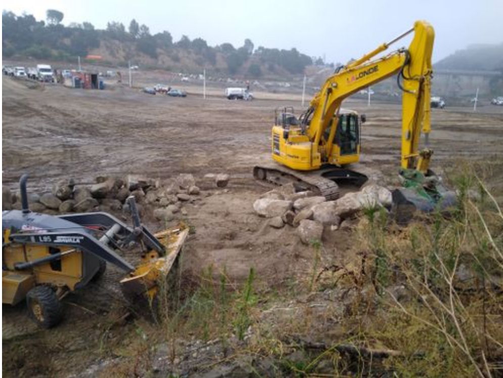
photo_1-excavator and skip moving boulders.jpg -118.17555 34.18966
