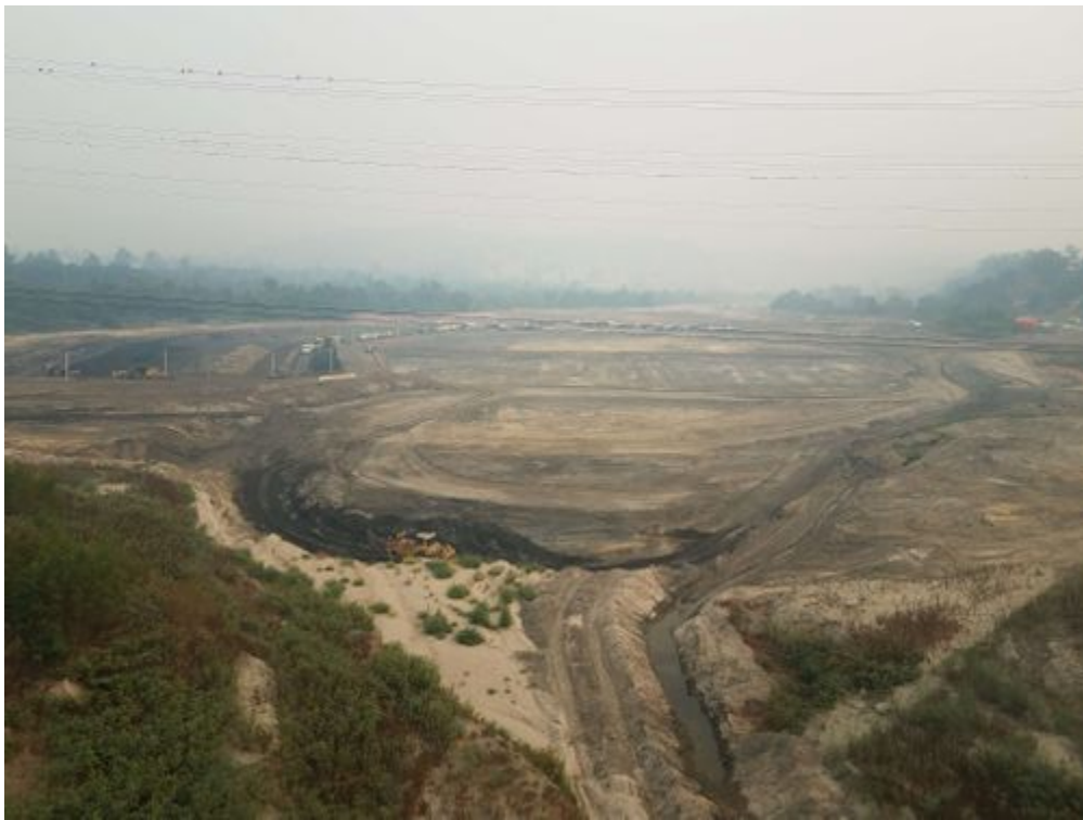
photo_4-20200915_site overview_facing N.jpg -118.17536 34.18532
