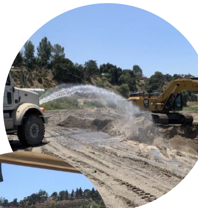
TOP: Water trucks watering sediment before being loaded into the trucks. BOTTOM: Watering all loaded trucks before leaving the reservoir.
