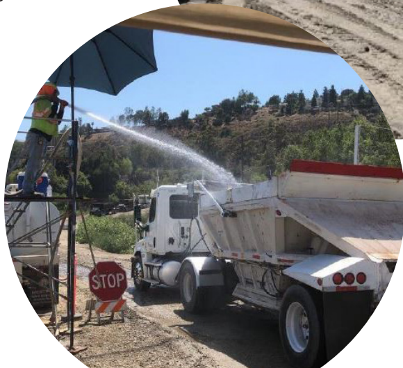
TOP: Water trucks watering sediment before being loaded into the trucks. BOTTOM: Watering all loaded trucks before leaving the reservoir.
